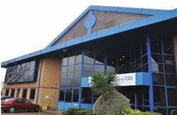
SITE ONE: CAHMS MENTAL HEALTH SITE (ONE ARMSTRONG WAY, WEST LONDON NHS TRUST)
